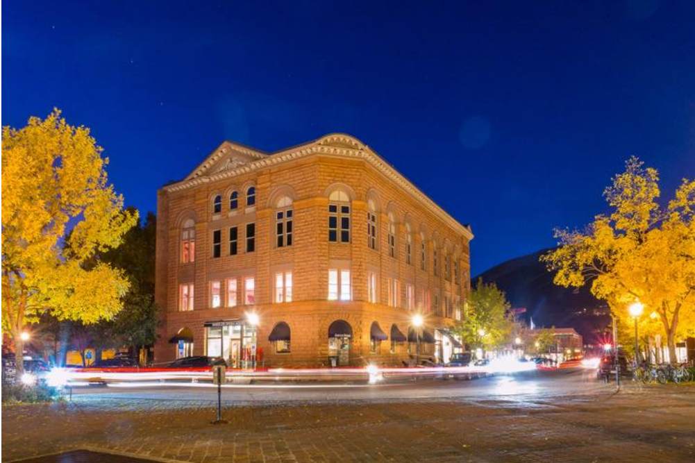
Wheeler Opera House Exterior
