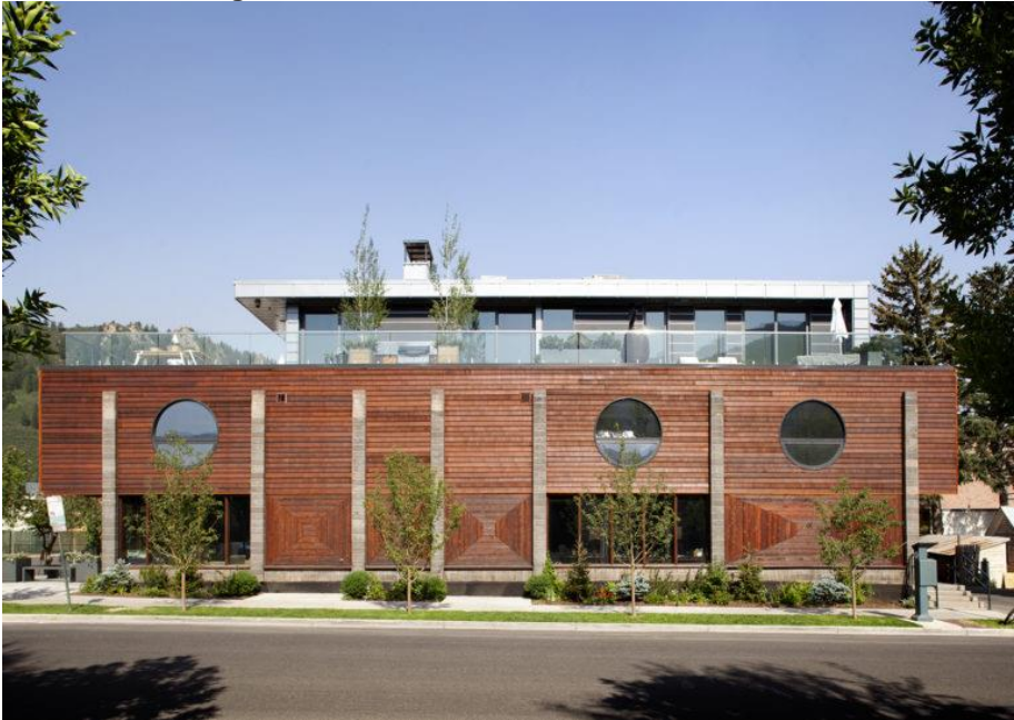
Crandall Building Exterior
