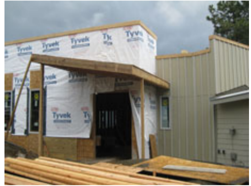
The addition in progress
