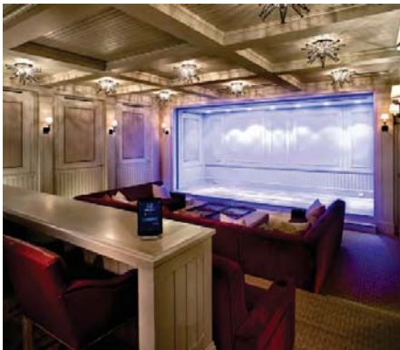
Lighting, heating, cooling, security, TVs, and speakers: In this McLain Flats home, everything is automated—even the shades! BELOW: Like most other components of the house, this home theater, installed by Xssentials at the Poss Architecture—designed Double Bar X Ranch, can be controlled with a single iPad.
